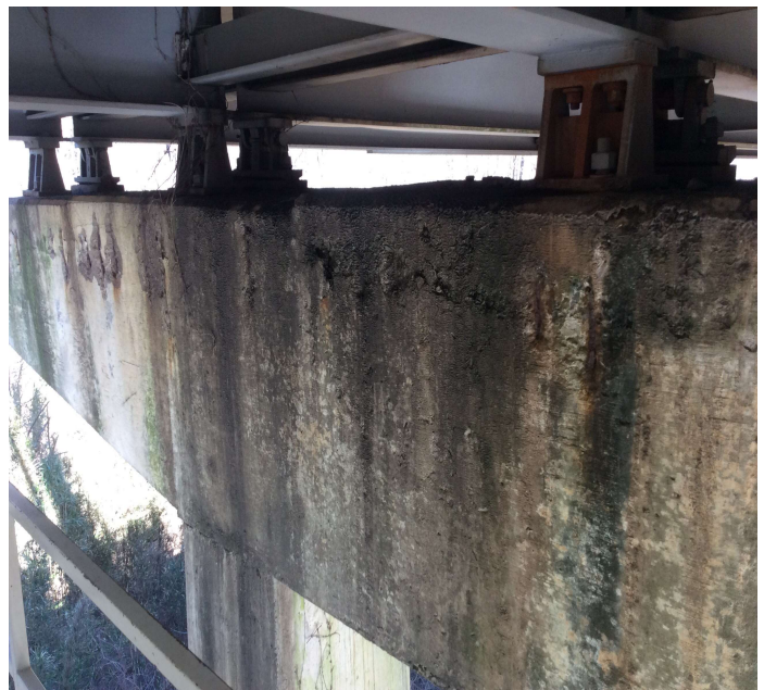
PHOTO 2 Description Delam, Cracking & Spalling W / Rebar Exposed in Bk. Face of Cap 5.
