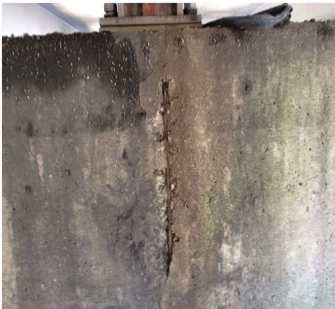
PHOTO 1 Description Typ. Delam, Cracking & Spalling W / Rebar Exposed in AHD Faces of Caps 6 & 7.
