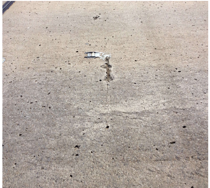
PHOTO 2 Description Minor Spall in Deck.
