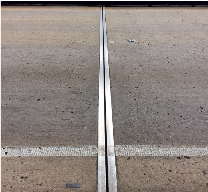
PHOTO 1 Description Seal missing at Joints.
