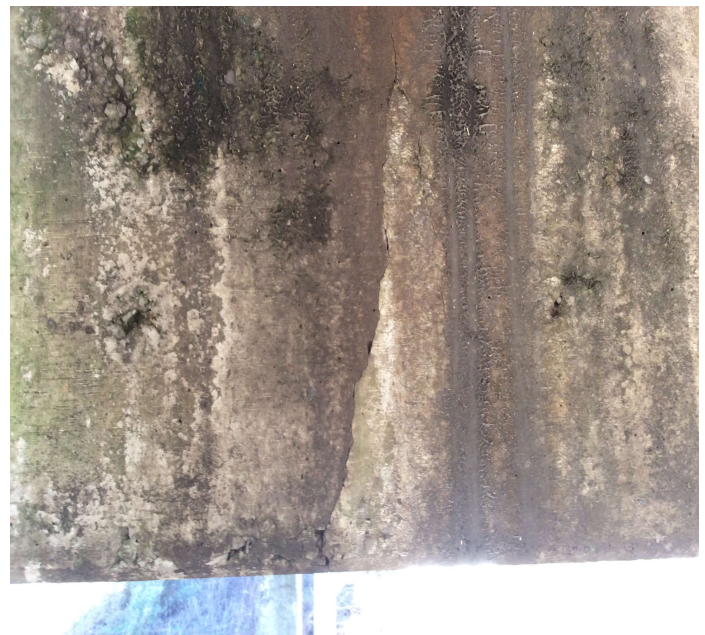
PHOTO 2 Description Vertical Crack in Cap 3 Bk. Side.
