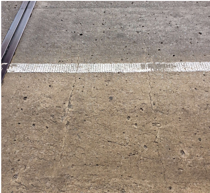
PHOTO 1 Description Typ. Cracking in Deck.
