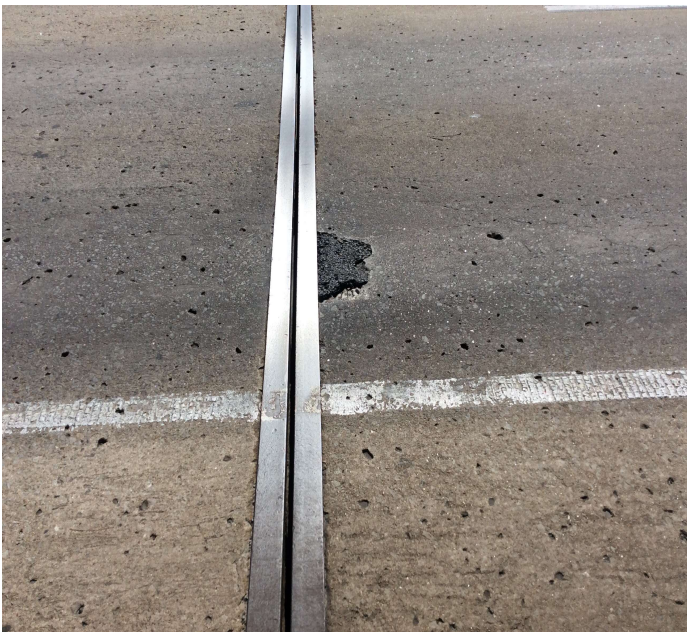
PHOTO 4 Description Typ. Minor Spalling at Joints 6 & 7.
