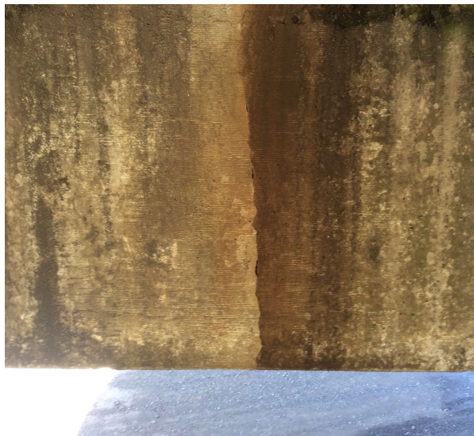
PHOTO 1 Description Vertical Crack in Cap 3 Ahd. Side.
